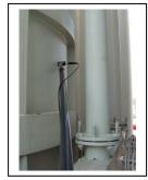
While the transformer tank vibration is being measured, the information is being stored in the device memory. The memory volume is enough for storing the data of 40 transformers' inspections. Later the data is uploaded to PC and is stored in «Vesta» expert software database.
