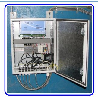
The «MDR-M» system is usually installed near the monitored electric motor, into the mounting case. The cable length from the PD sensors to the device should not exceed 50 meters.
